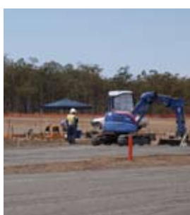
Foundations being laid
