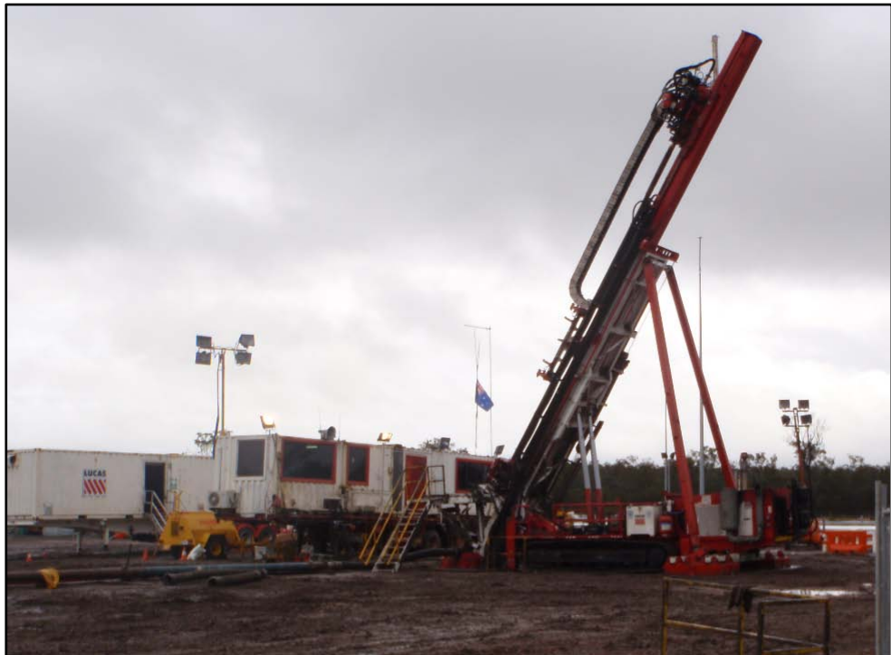
Horizontal drill rig for Panel 2
