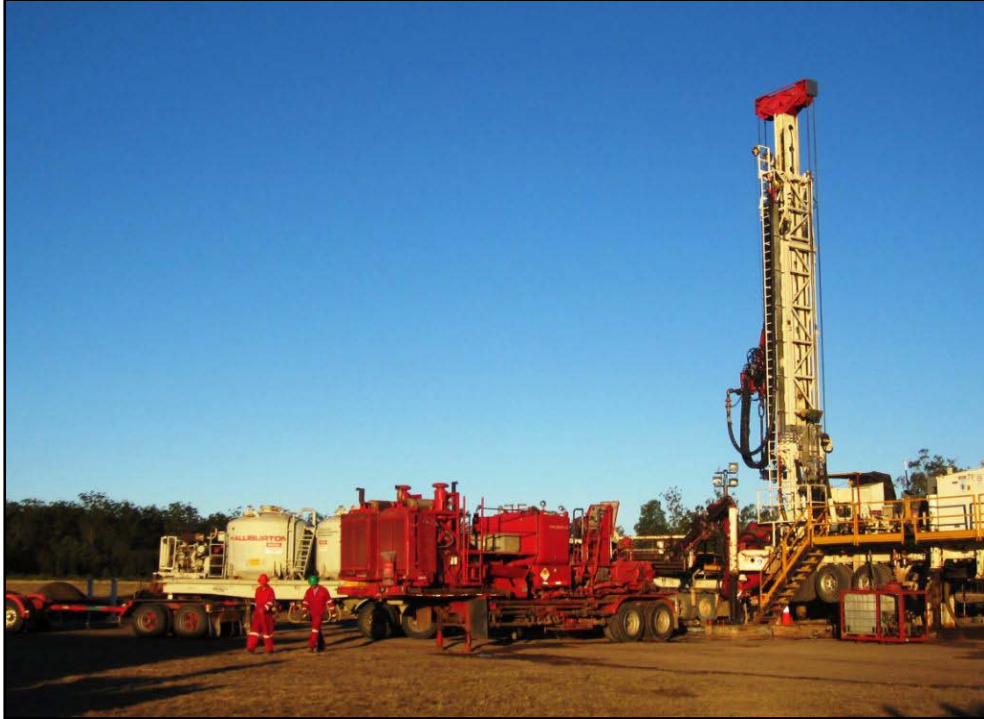
Vertical drill rig for drilling of Panel 2
