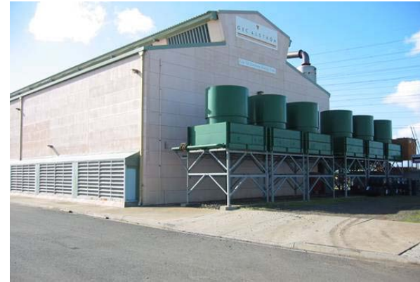
Existing generating station, Sunshine
